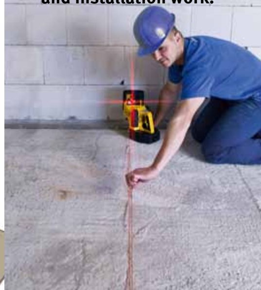
LA 180 L: 3 vertical lines, 1 horizontal line and plumb function.
